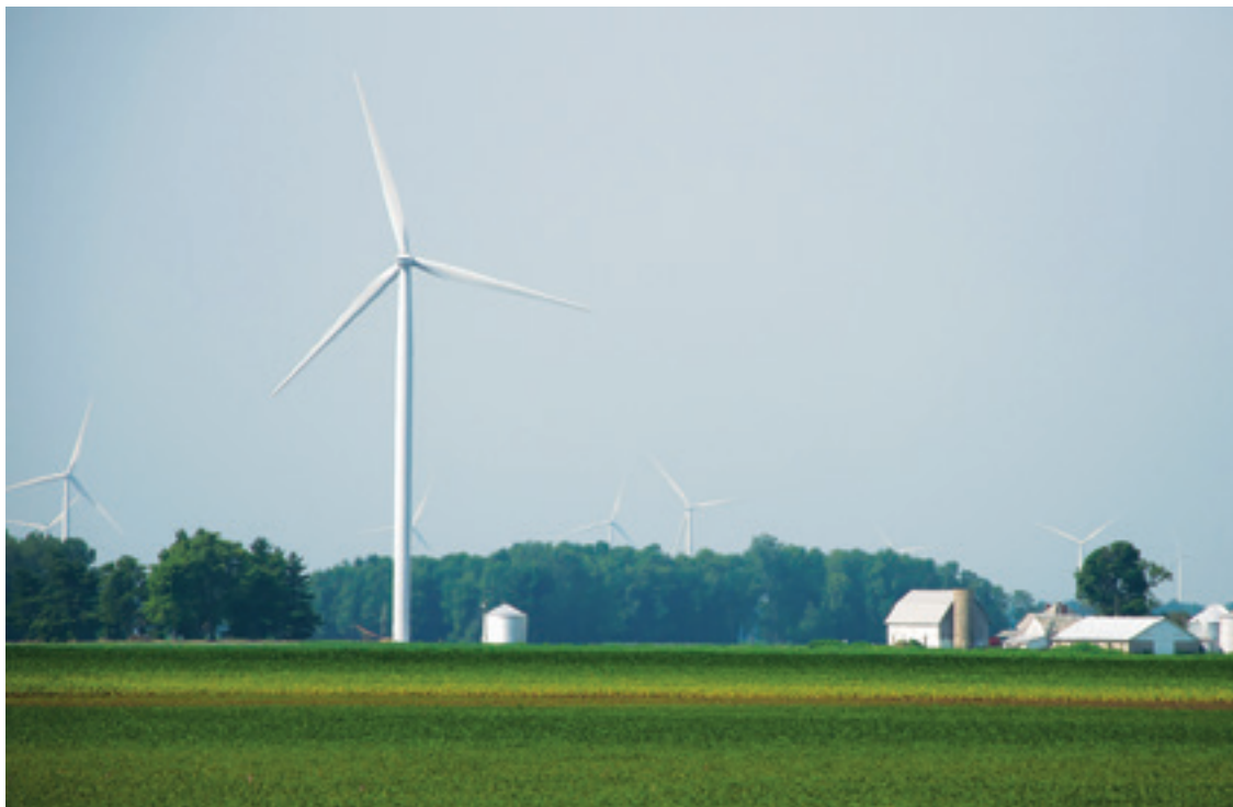
Figure 8-5. GE 1.6-MW wind turbine. German utility E.ON installed 125 of GE's 100-meter (328-foot) diameter turbines in the first phase of its Wildcat Wind Farm near Elwood, Indiana. With a specific area of 4.9 \text{ m}^2/\text{kW} —about twice that of wind turbines manufactured only a decade before—GE's 1.6-MW wind turbine has been designed for areas with low to moderate wind speeds. 2013.
