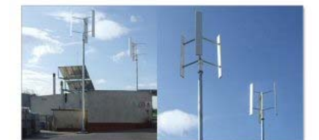
Installation at Sligo, Ireland - V3.5 Installation at Sligo, Ireland
