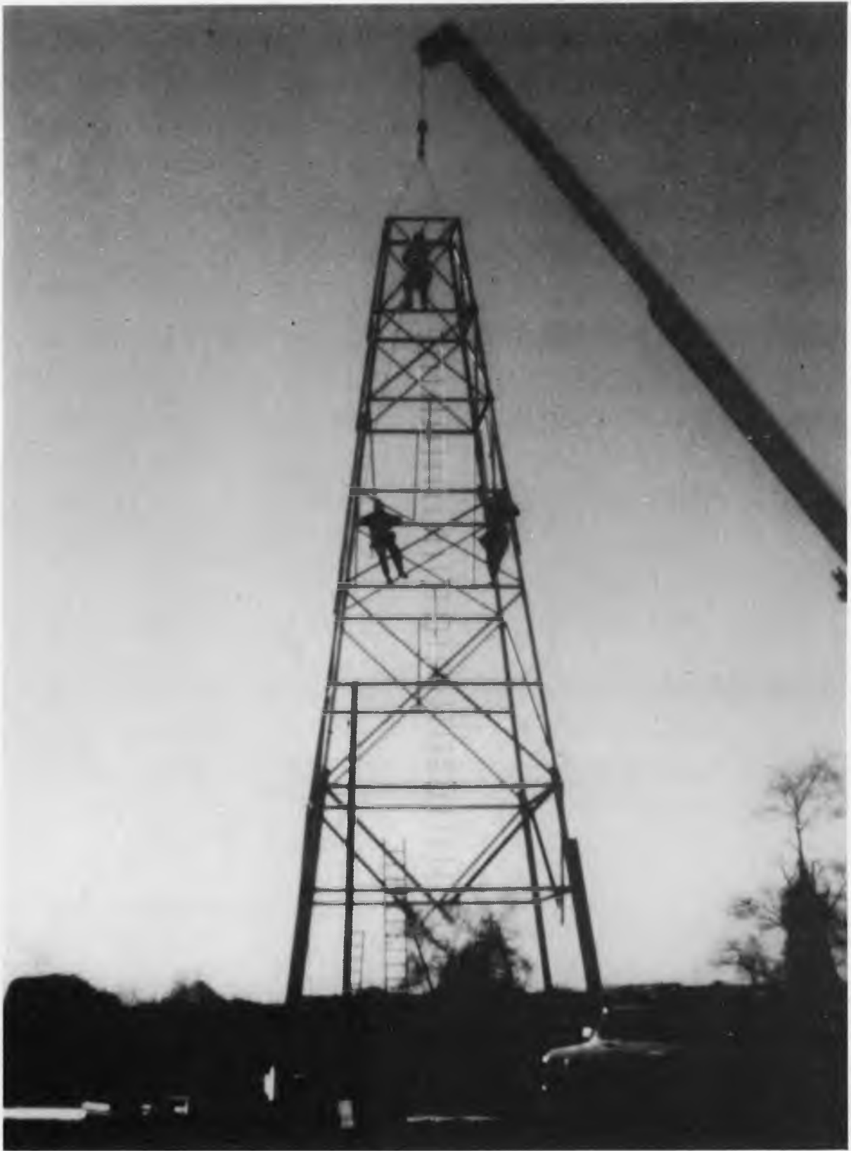
FIGURE 17 FIXED TOWER AFTER INSTALLING THE UPPER SECTION
