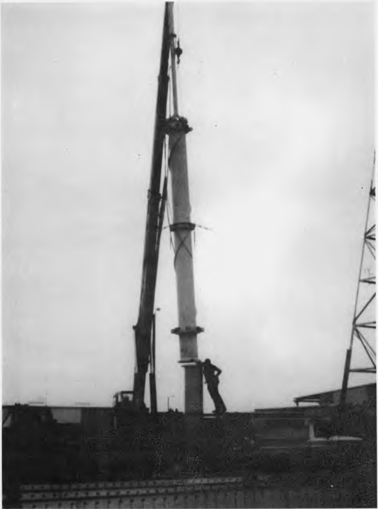
FIGURE 19 ATTACHMENT OF ROTOR TO ASSEMBLY STAND
